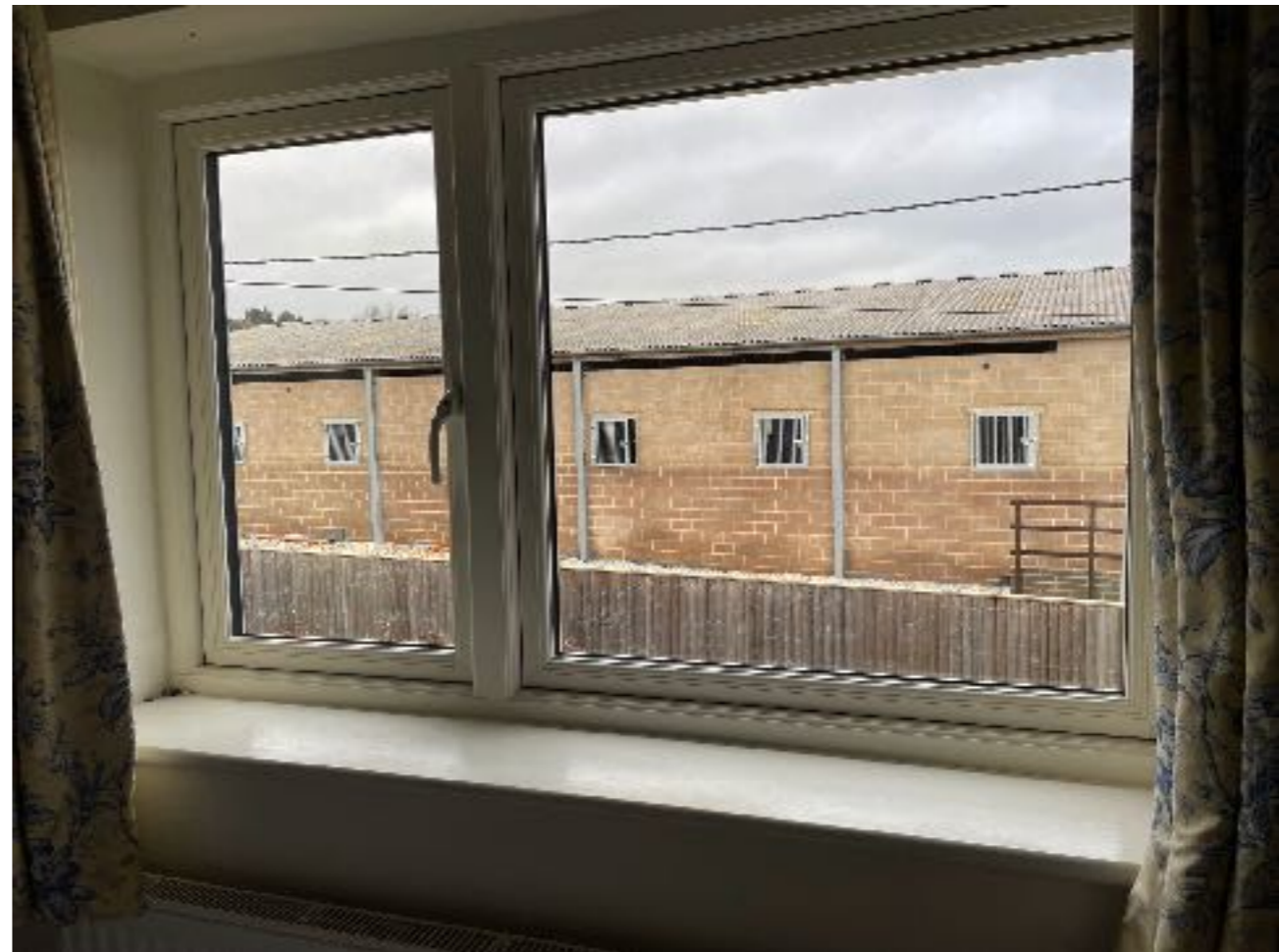
windows/tackroom ramp from first floor main bedroom
